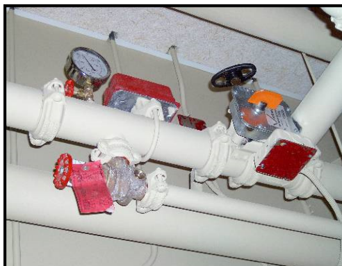
Image 3 – Sprinkler Flow Switch and Control Valve c/w Tamper Switch
