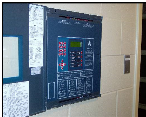
Image 8 – Fire Alarm Annunciator Panel – Main Entrance on Main Level
