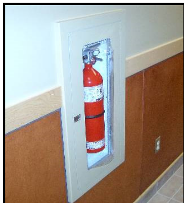
Image 11 – Portable Fire Extinguisher in Cabinet
