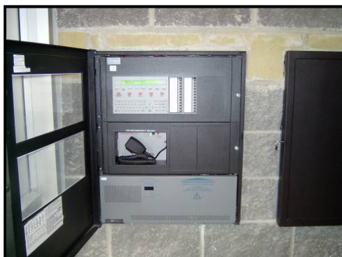
Image 6 – Main Fire Alarm Control Panel
