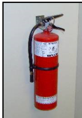
Image 12 – Wall Mounted Portable Fire Extinguisher
