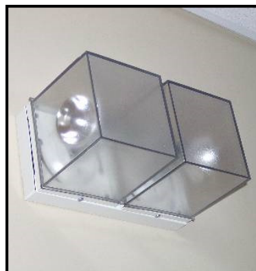
Image 14 – Emergency Lighting Unit Lamps
